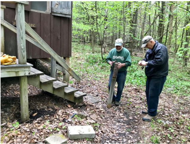
Brion and Gary work on replacing an existing staircase railing
